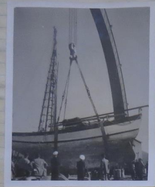
Hoisting out at Sumatran
